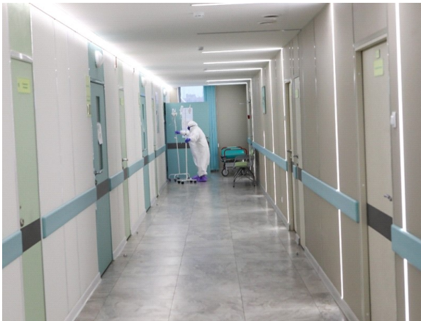
Internal wall Cement Board
